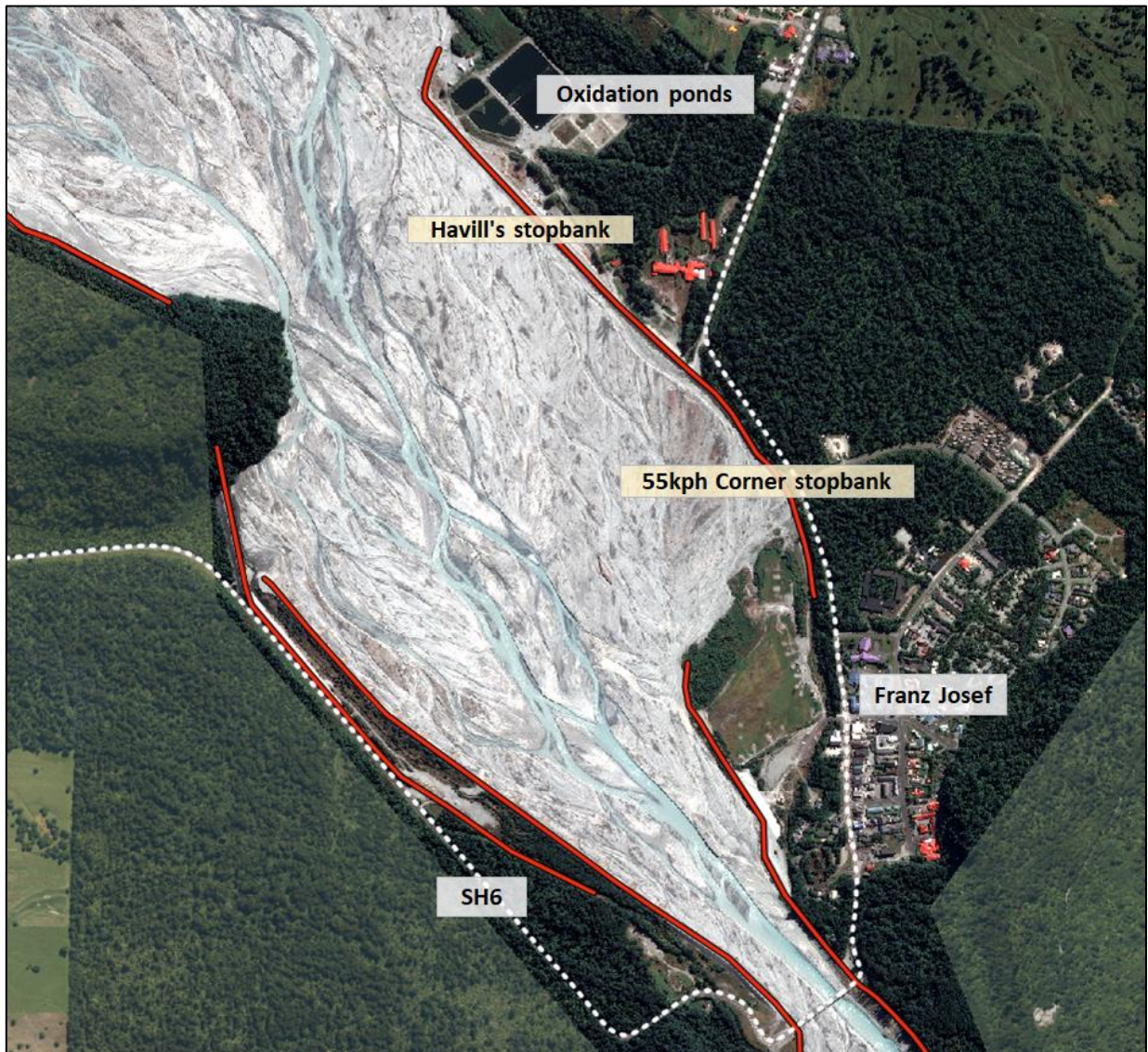
Figure 3-8 – Aerial imagery from 2021 showing the Havills and 55kph corner stopbanks.
