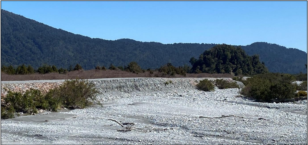
Figure 3-10 – An unlined section of the Rubbish Dump stopbank between Canavan's Knob and Rata Knoll.
